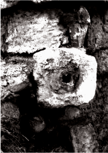
Ancient water pipe clogged by mineral deposits.
